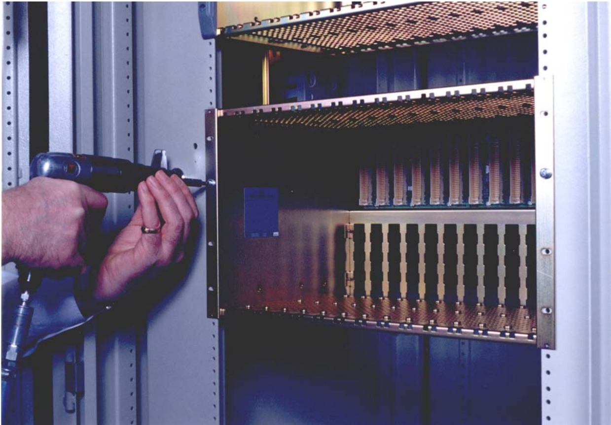
Figure 4-3: Controller Chassis Installation
